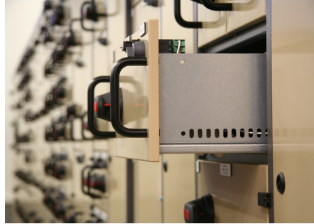
PICTURE: Cassette is drawn out into the separating position. It can be fully taken out by releasing the separation latch.
